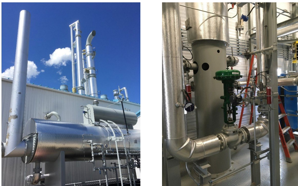
FIGURE 2. InnoTech-ASCO/HTC CO 2 Capture System Hot Oil Supply, Adsorber, and Stripper Columns (L) and Stripper Column (R)
